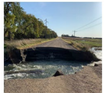
Figure 2. Work in water due to a road collapse may require US Army Corps of Engineers NWP or 401 or 404 depending on the method of repair. FEMA photo.
